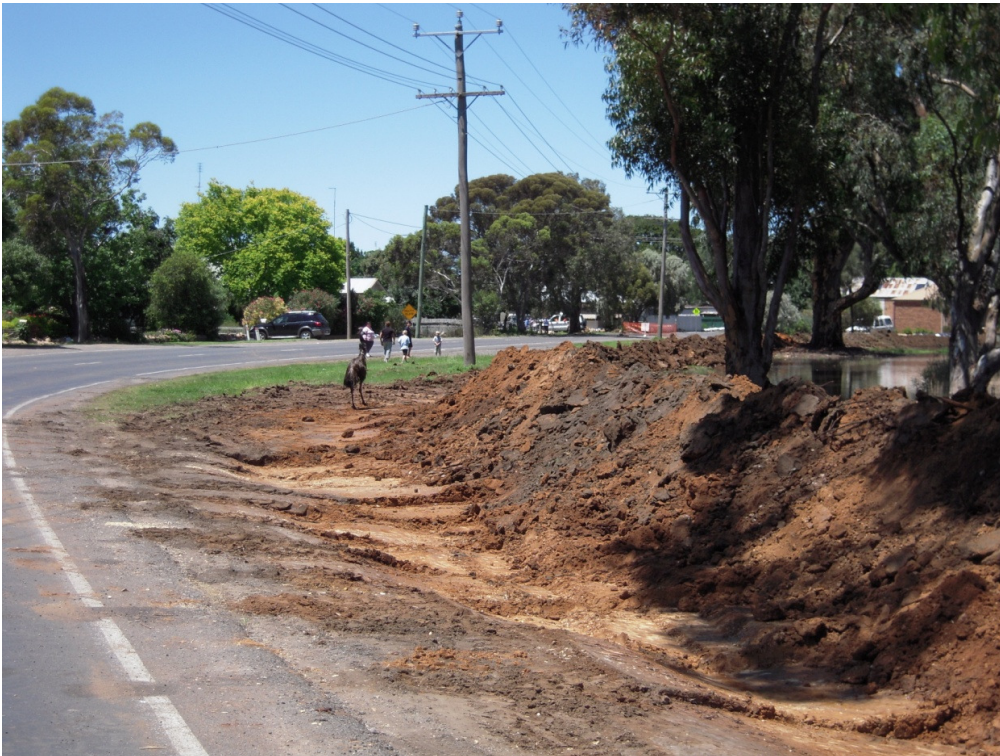
Figure 4: Informal embankment along Yarriambiack Creek in Warracknabeal. Note it has artificially raised the water level on the right-hand side.
